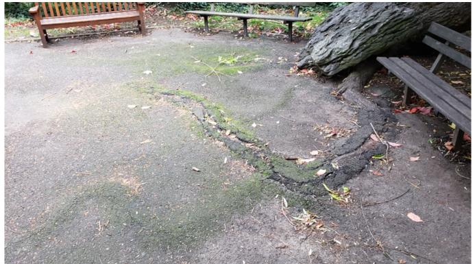
Note the roots pressing up against the paving highlighted by the moss overgrowth. Here's a snap showing the rock laid across the base of the tree:
