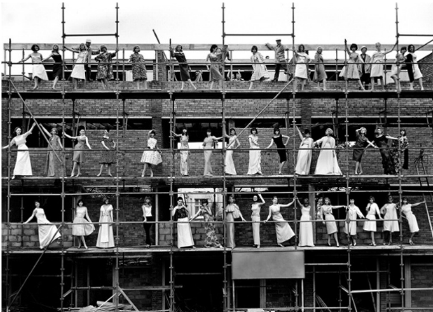
Models on scaffolding, London 1977
